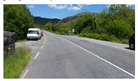
Upon reaching Clonkeen to the North, the road terminates and joins the N22. The road is a marked two-lane road with a good metalled surface, suitable for supporting the vehicles utilised for the transportation of construction materials. The signage that is visible in the above indicates the turn from the R569 at Morley's Bridge, corresponding with the beginning of the L3021.
