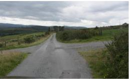
Certain parts of this section of road are wide enough to accommodate a single lane closure for construction of the UGC, while allowing room for cars to pass, using either traffic light signals or stop and go men.
