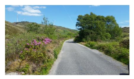
The remainder of this section of the road could be classified as fair to good. There is no public transport or pedestrian pathway on this road section. The speed limit is posted as 80 km/h.
